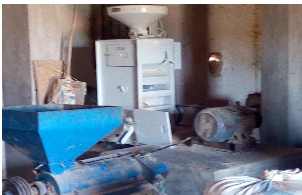
Example of a small two step mill in Butaleja.
